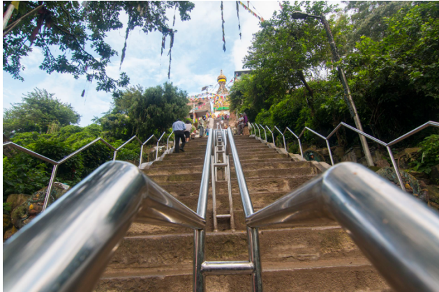
Eastern Staircase from Wikipedia 2023
